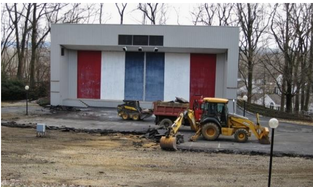
Impervious Asphalt Being Removed at the Amphitheater
