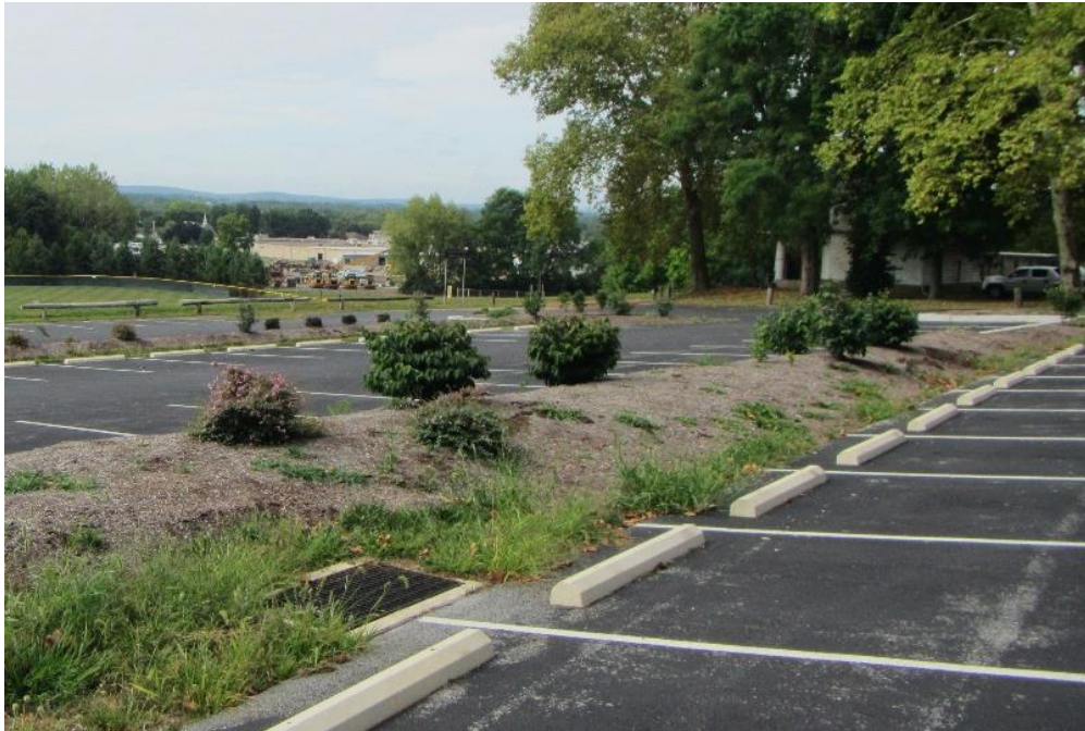
Islands in Parking Lot Infiltrate and Collect Stormwater For Irrigation of Adjacent to Sports Fields.
